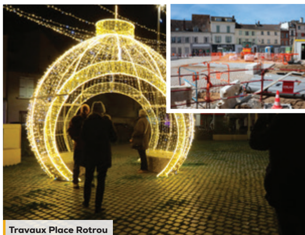
Travaux Place Rotrou
